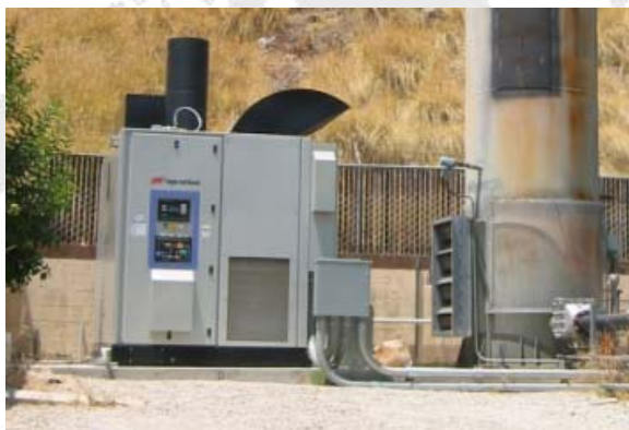
250 kW microturbine at Burbank Landfill
